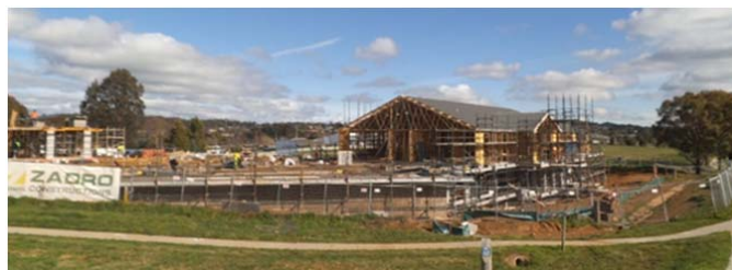
Construction of the Columbia Homes Aged Care Facility
