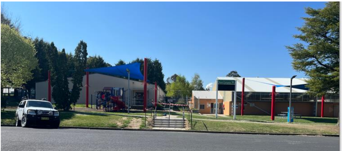
Figure 3, Street View of Gym and Pool facilities
