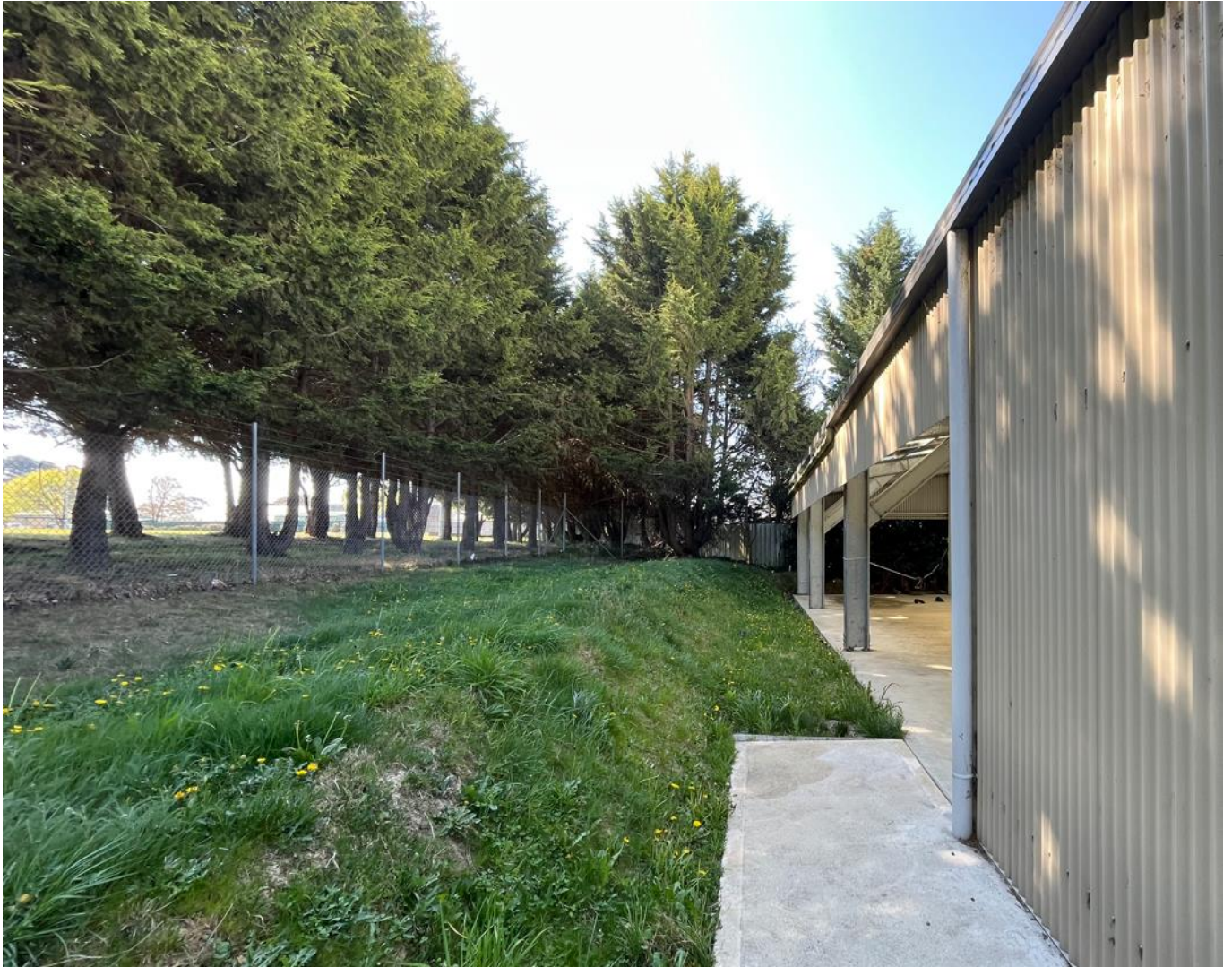
Photo 3: Rear of Northwestern elevation showing connection to adjacent football field.
