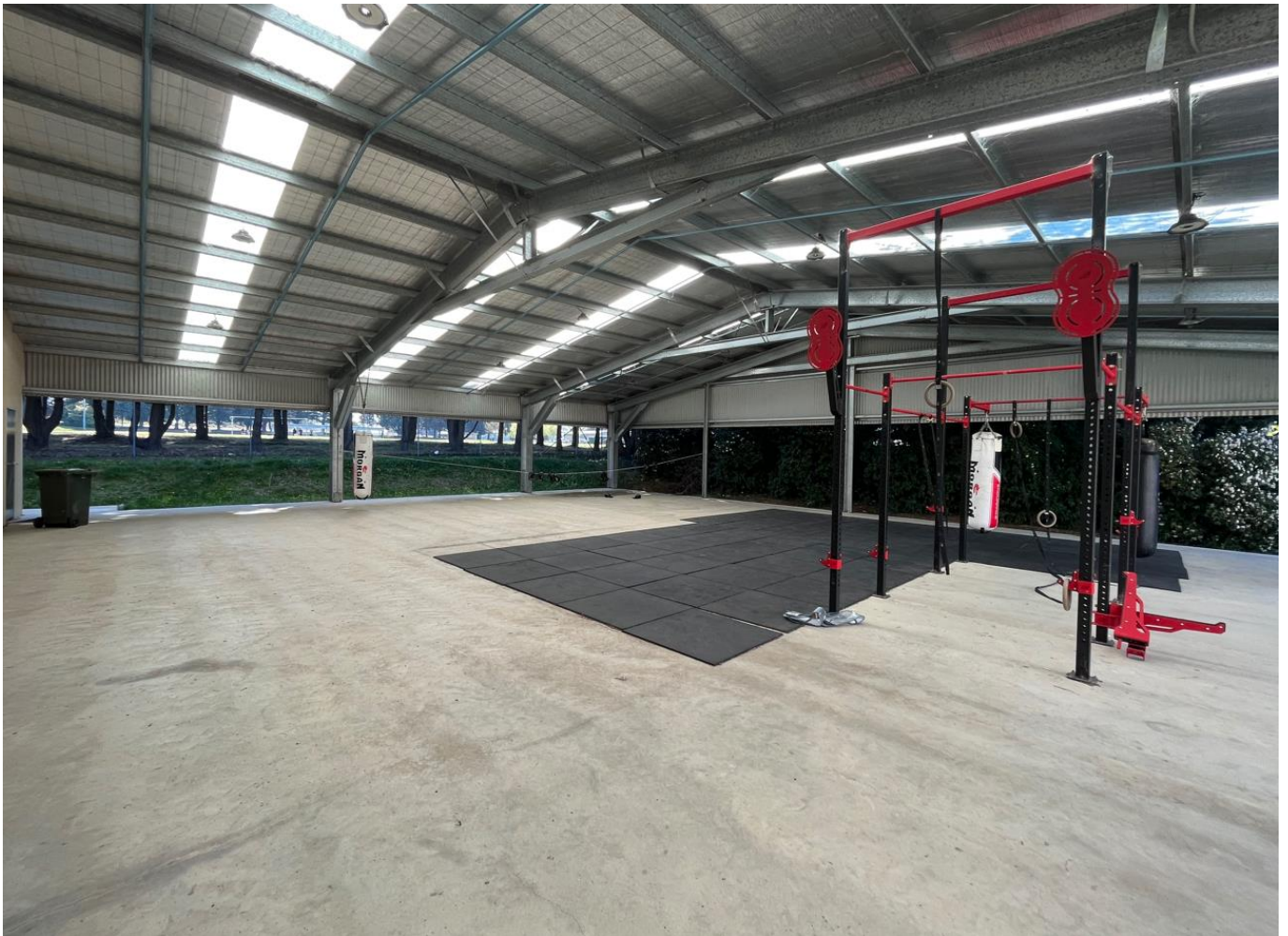
Photo 4: Internal space to be enclosed
