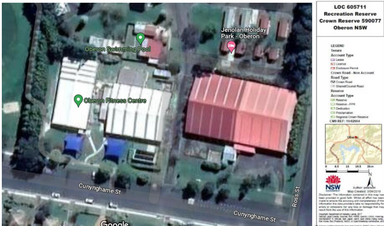
Figure 1 Existing building in the context of the site.
