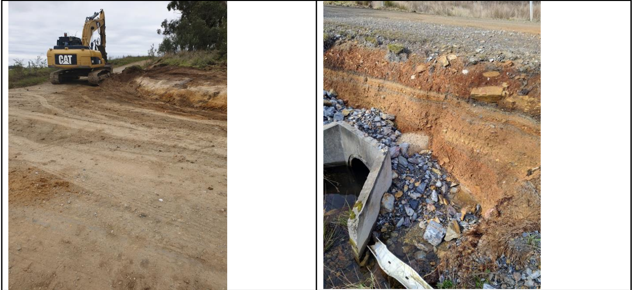
Figure 4: Culvert replacement of culver on Beaconsfield Rd and repairing of scouring behind headwall on Jaunter Road.
