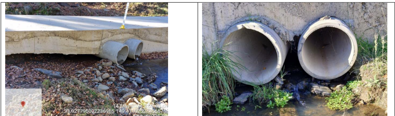
Figure 5: Significant scouring has resulted in lowering the load limits for Bald Ridge Creek and Unnamed Creek crossings to two tons.
