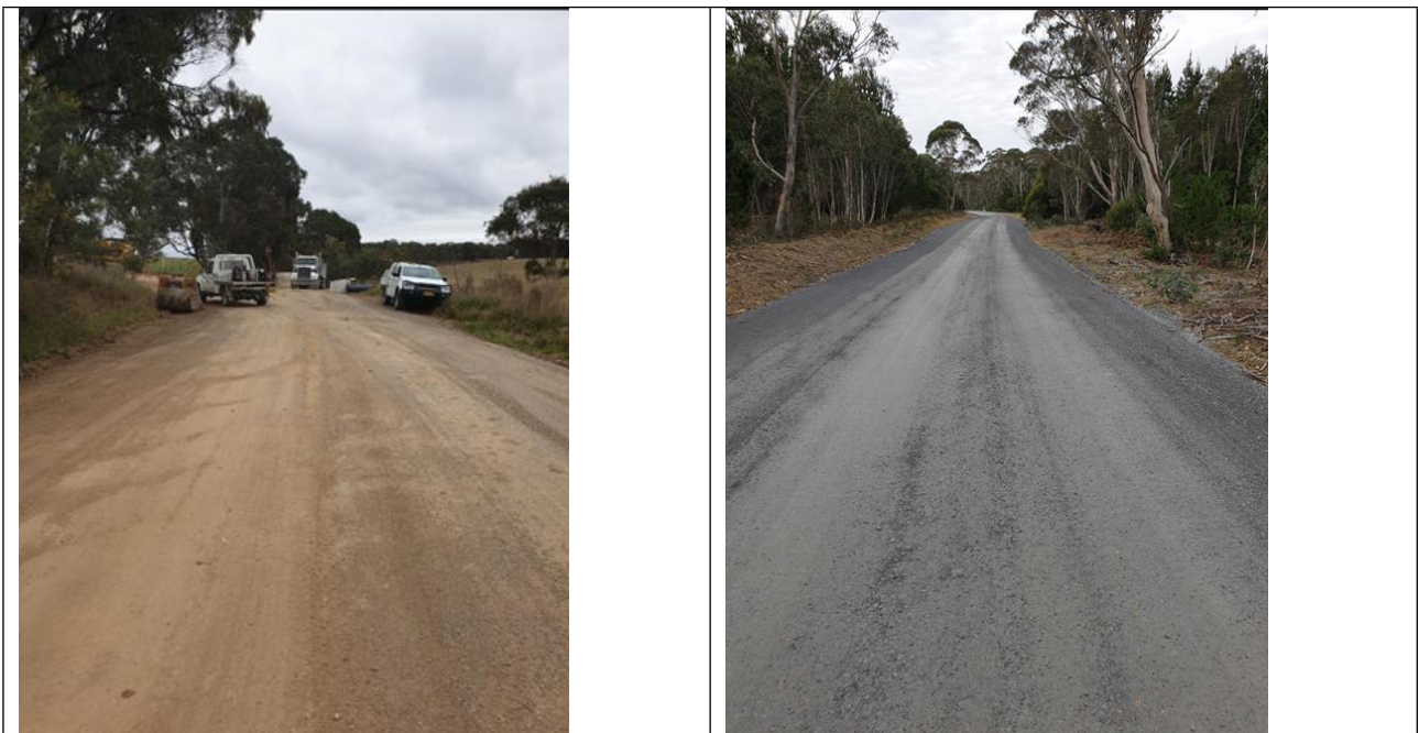
Figure 3: Road gravel re-sheeting works on Beaconsfield Rd and Bastards Point Rd
