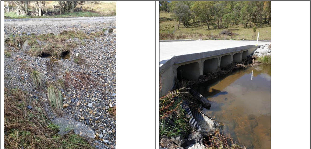
Figure 2: Severe silting of drains on Springmount Rd and pipe culvert at Nunan's Hill bridge.
