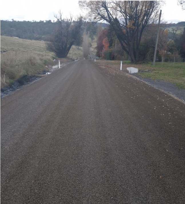
Figure 3: Seal on Nunan's Hill Rd for erosion control
