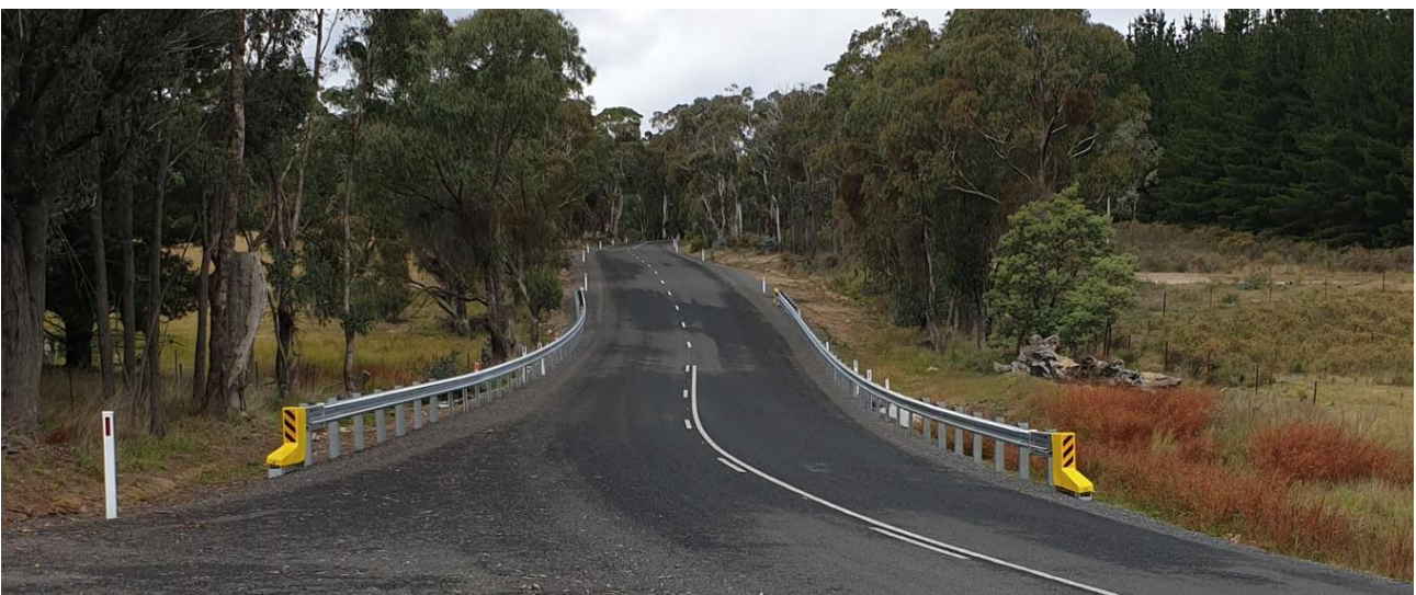
Figure 1: New guardrail on Arkstone Rd
