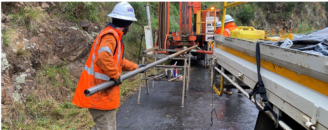
Drilling investigation work at Five Mile
